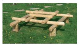
Glue notch joints on (B) and build the frame back up. Slide the sections around until you find best fit. Using a drill, screw up tight with screws provided while placing downward pressure.
